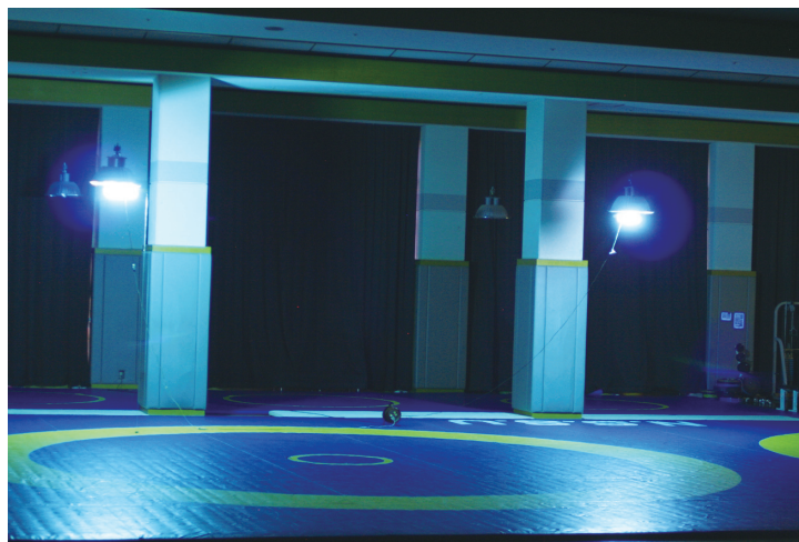
Fig. 3. The ultraviolet irradiation in wrestling facility. Figure shows the ultraviolet-lamp from the 3 meter height irradiated to the wrestling mats and floating microorganisms.
